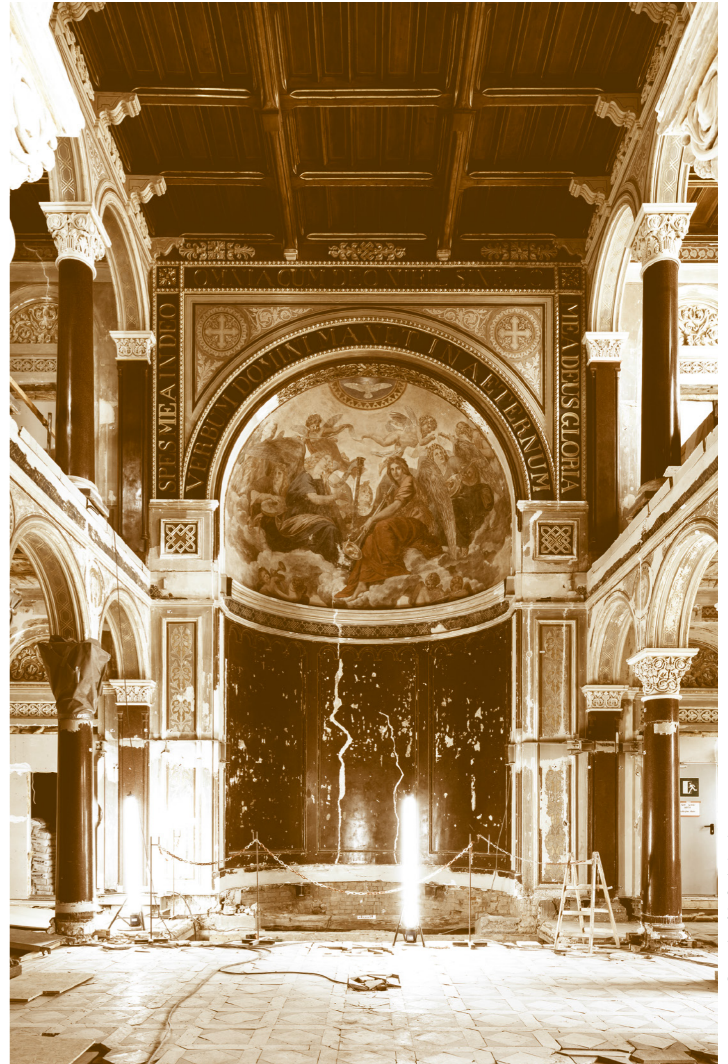
Restoration of the Castle chapel
